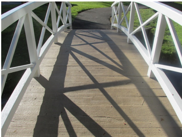
Bridge deck boards
