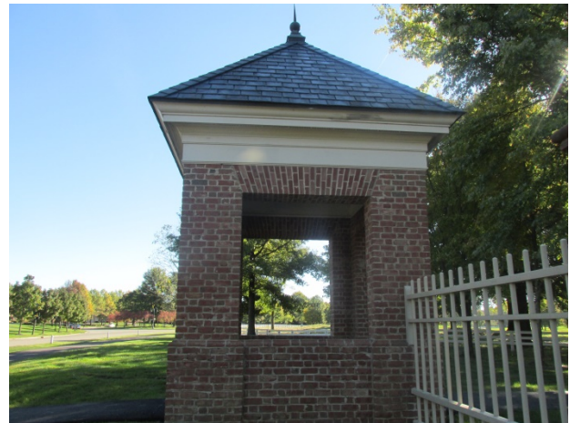
Masonry framed gazebo
