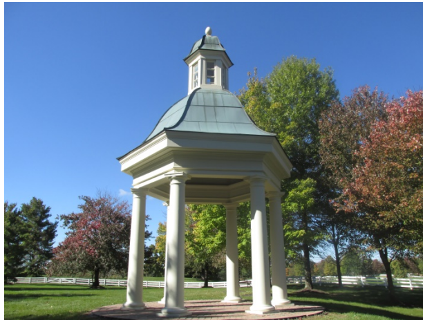
Wood frame gazebo with wood metal roof
