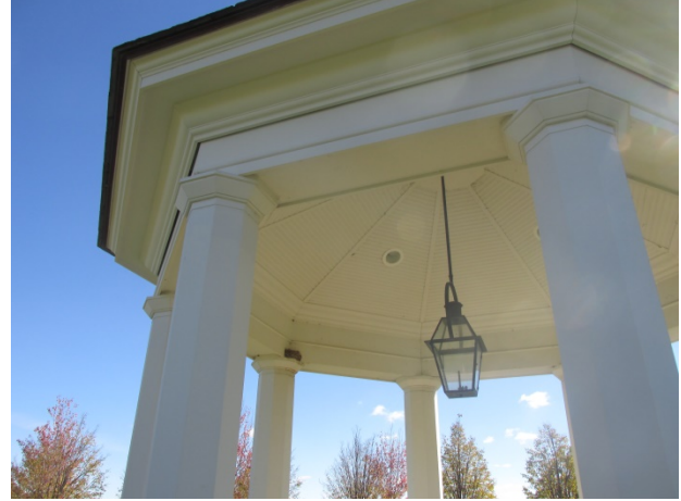
Structure and light fixture at gazebo
