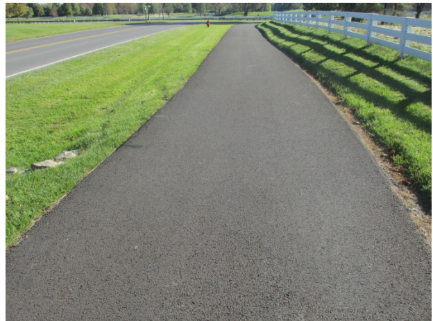
Previously replaced asphalt pavement walking path
