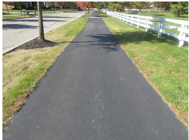
Asphalt pavement walking path at Southfield
